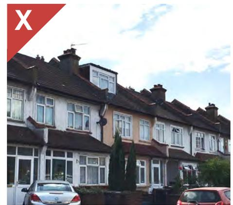
Figure 4.21f: Example of an inappropriate addition of a front dormer to a mid-terrace house. This addition lacks design merit and breaks the uniformity of the roofs that contributes to the positive characteristics of the street.
