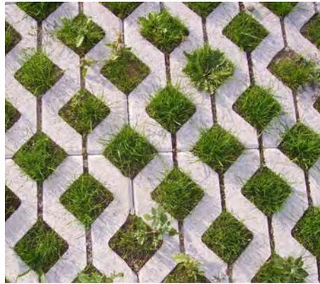
Figure 2.36e: Permeable paving.
