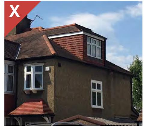
Figure 4.21e: Example of where a side roof extension to a house has not been setback from the original roof. In this situation it has compromised the symmetrical form of the original semi-detached houses and therefore negatively impacts the appearance of street.
