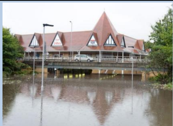
Figure 1 Purley Cross underpass (Croydon, 2015)
