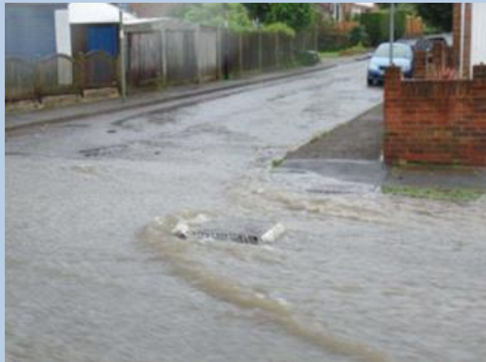
Figure 3 Surcharging manhole on Caterham Drive
