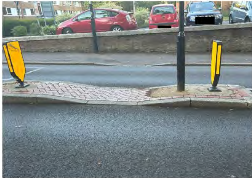
Photo 2: Existing Central Island
